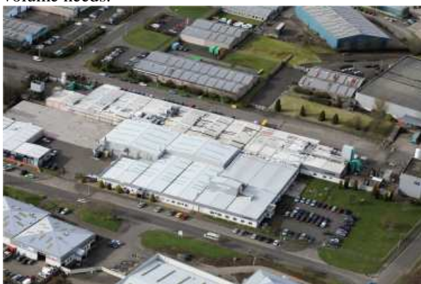
Figure 1 - Aerial View of Semefab, Glenrothes, UK
